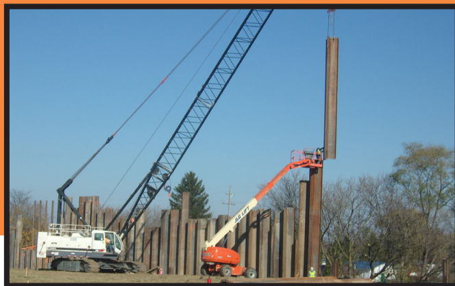
Sheet pile wall being installed. See page 1 for more information.
